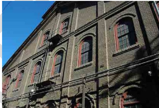
The existing Central Shops in the Railyards Plan Area.
